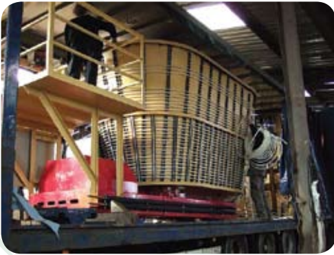
Image: Construction of innovative pre-digestion equipment in Omagh
